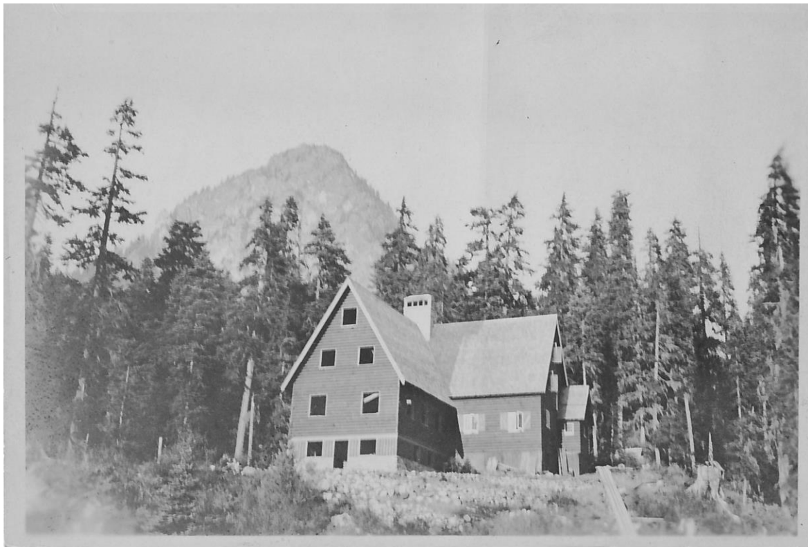
The original Commonwealth Ski Club lodge under construction in the summer of 1932. (Photo from the Mahnken family collection.)
