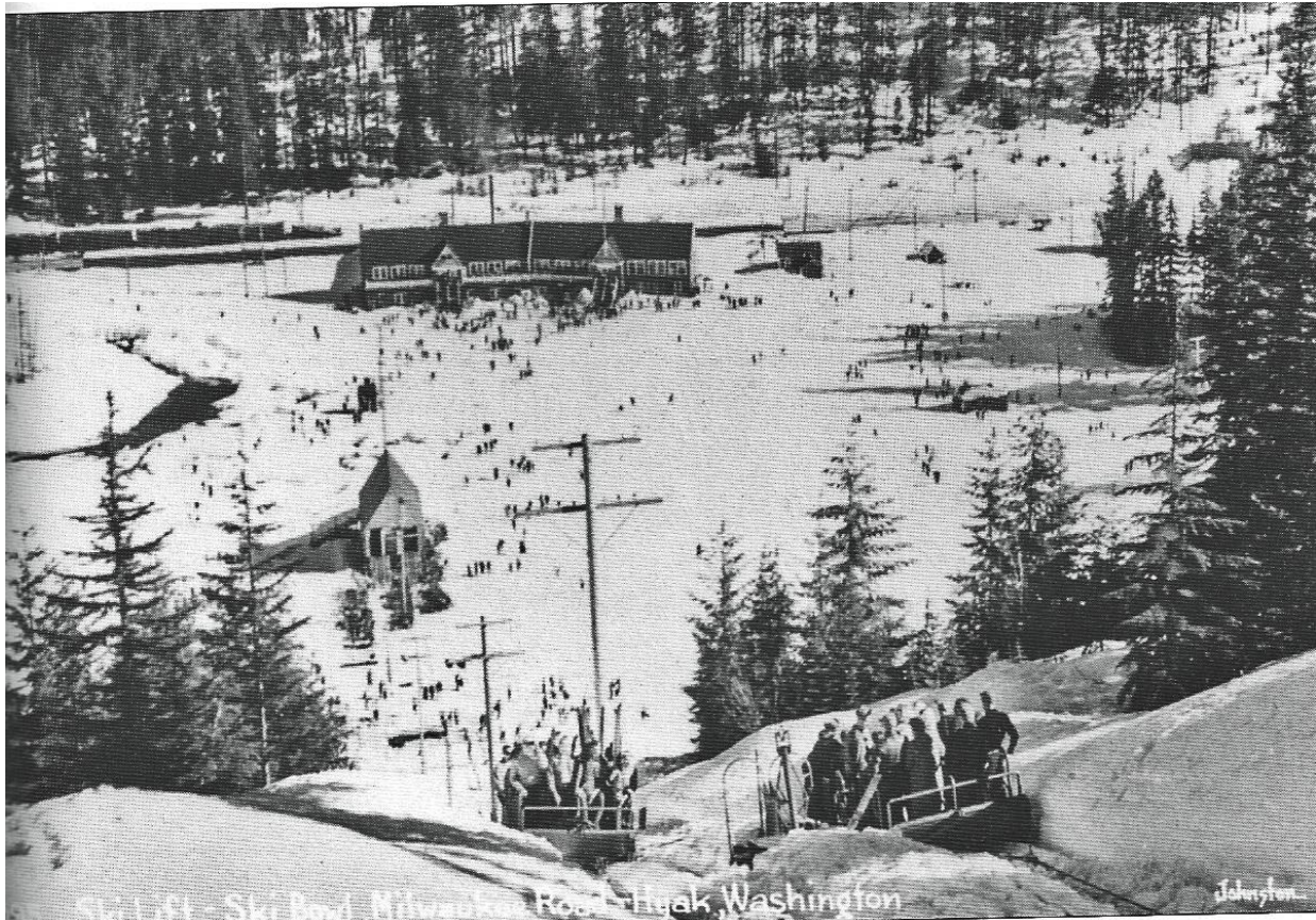
Figure 4. Photo of the Tally-Ho Skiboggan at the Milwaukee Road Ski Bowl c. 1947. The up sled is on the left (note skis being carried up), while the down sled is to the right carrying sightseers. (Photo by __ Johnston, from the collection of Jack Leeper.)
