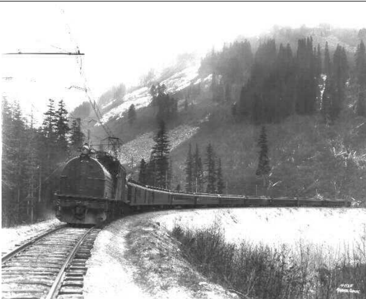
Photo by Asahel Curtis, c. 1925, entitled, "Milwaukee Road Electrification: Passenger Train showing trolley construction, Cascade Mountains, Coastal Division," borrowed from "Dave's Electric Railroads" website, http://www.davesrailpix.com/cmstp/milw.htm , accessed 10/21/2011.
